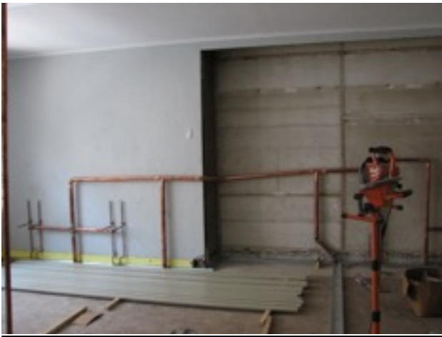
Figure 2 Old Nursery, showing roughed-in plumbing for new restrooms
