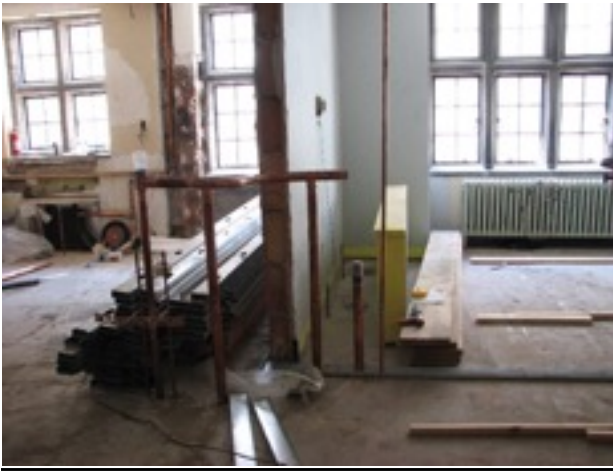
Figure 1 Parish house merged old women's restroom and kitchen showing roughed in plumbing.
