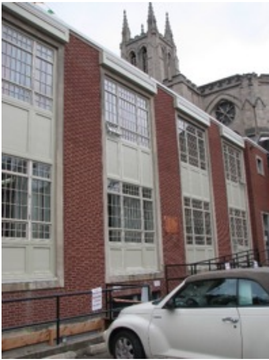
Figure 7 West Wall, Pennington Center showing new windows, Hardie board below windows and top decorative filler. Note also the top decorative element that is a new addition to design.
