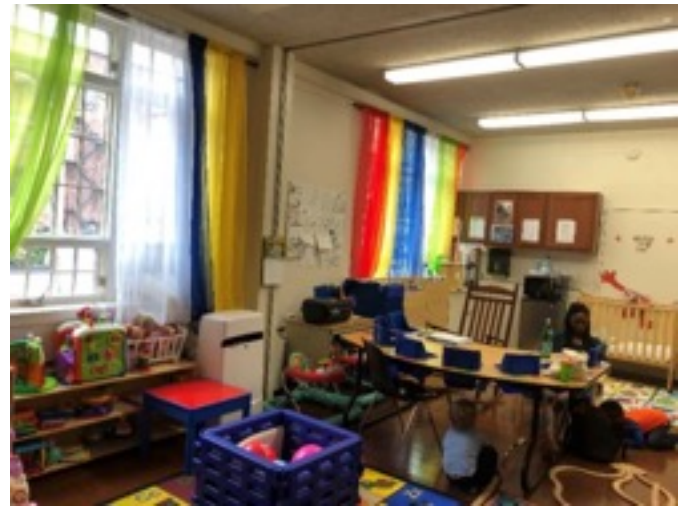
Figure 9 Interior of nursery room. New windows installed and new exterior wall modified to add insulation.
