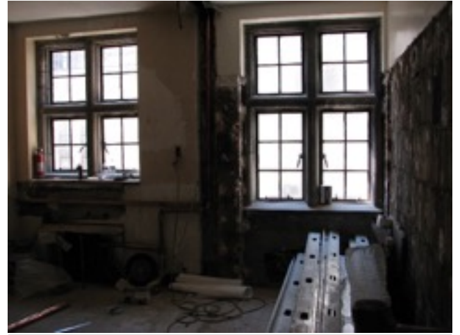
Figure 4 Wall removal: Old Women's restroom and Kitchen area.
