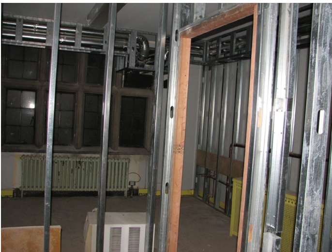
Figure 10. View into new bathroom and lounge area.
