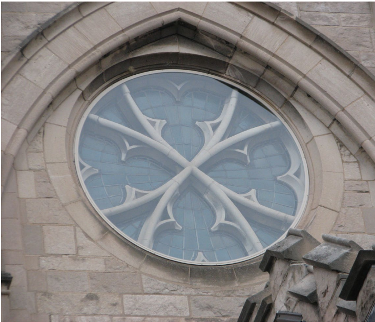
Figure 4. Round window from outside showing new storm window
