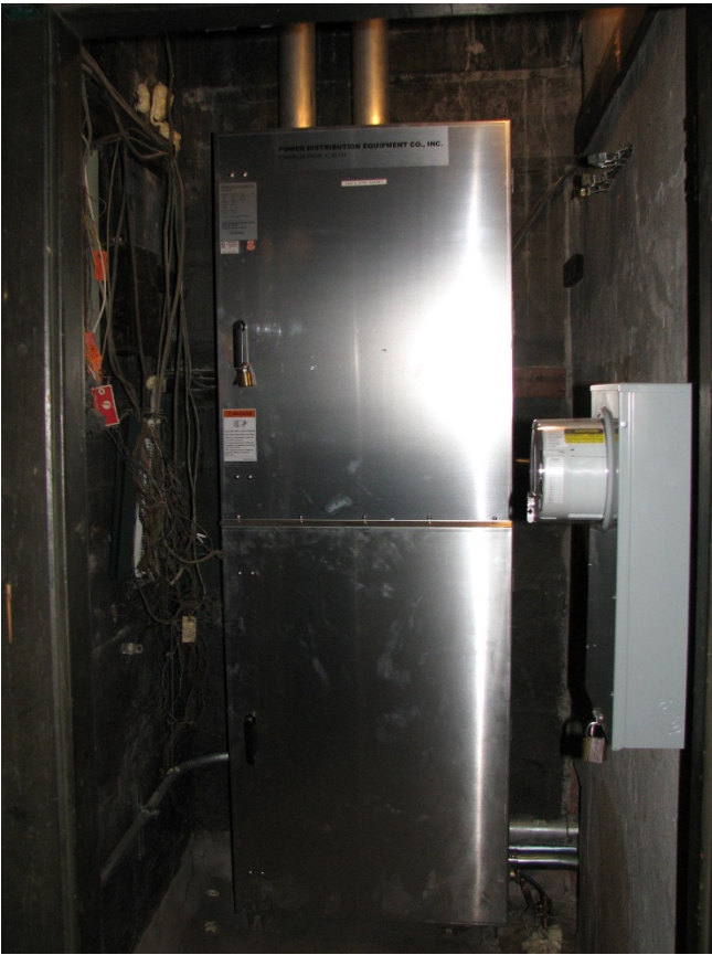
Figure 12. New building power feed for all buildings.
