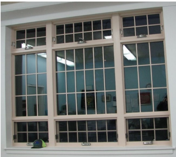
Figure 2. Interior of new Pennington Windows in Volunteer Office
