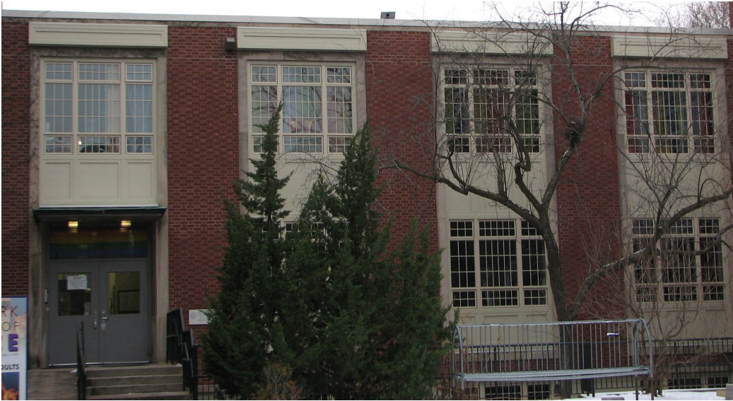
Figure 1. Front of Pennington Showing new Windows installed.
