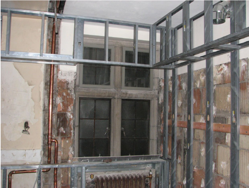
Figure 8. New Kitchen area. Windows out onto alley.
