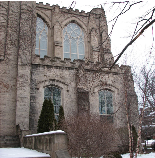
Figure 6. South facing window of Sanctuary and VOV.
